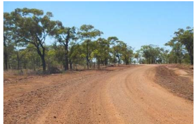
Gregory Developmental Road following completion of reconstruction works after 2014 event damage
